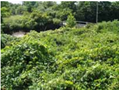
Maple Beach Bridge over Otter Creek
