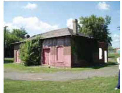
Abandoned Water Department Shed near Marsh
