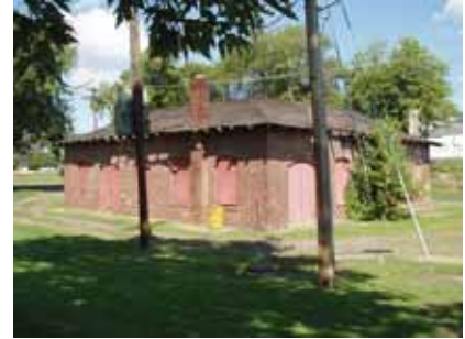
Abandoned water department shed near Marsh
