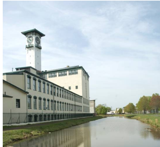
Grundy Mills along Delaware Canal
