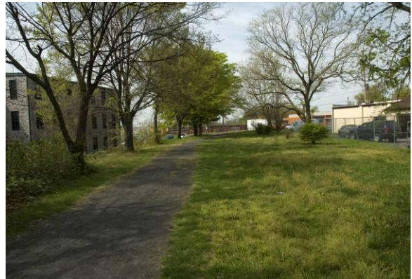
Filled Portion of Delaware Canal behind Canal Works
